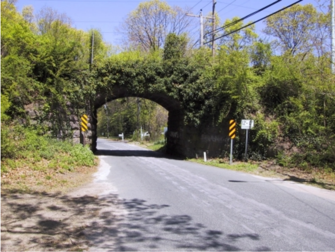
Figure 4. The LIRR Bridge
