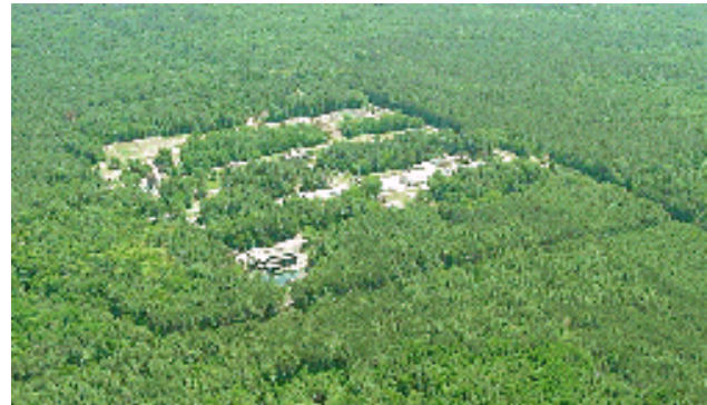
Figure 14. Saratoga Technology & Energy Park, Malta, NY
